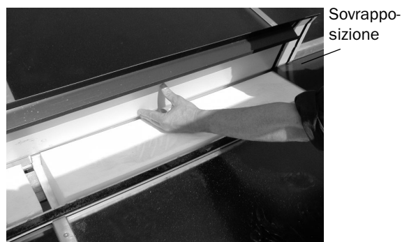
Fig. 108: Applicare le lamiere intermedie
